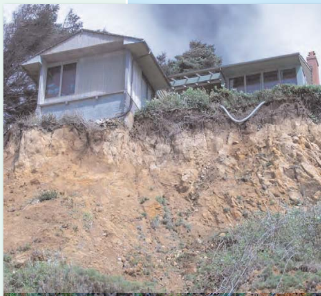
Chronic erosion and landsliding along Cove Beach, near Cape Falcon, has required many homeowners to modify or move houses away from retreating sea cliffs.
