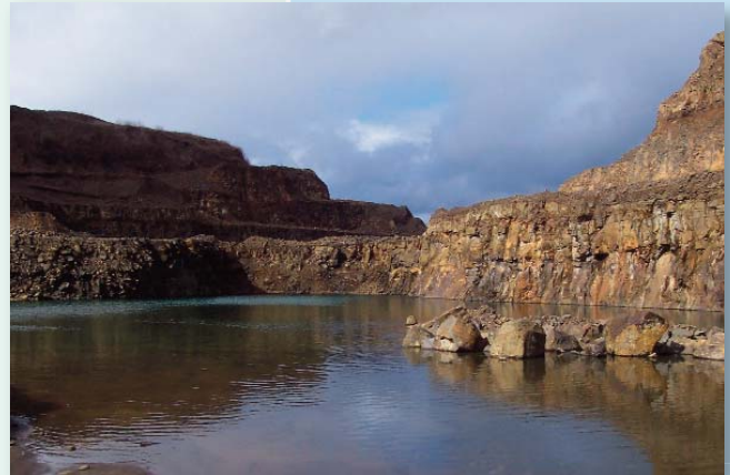
The 80 acre Beaverton Quarry has an effective stormwater control system and concurrent reclamation is being practiced on mined-out areas.
