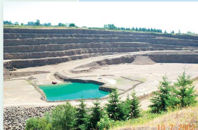
Concurrent reclamation continues to be practiced, with overburden from new areas spread over mined out areas and revegetated, thereby limiting the overall area of disturbance.
