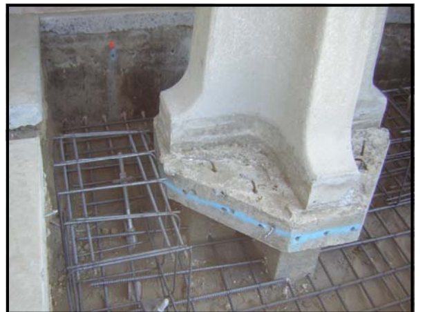
Figure 2. Construction process used for installation of helical soil anchors (A) surrounding soil excavated around the column (B) helical soil anchor installation (C) proof testing helical soil anchor (D) compaction of soil surrounding the column (E) drilled holes for installation of epoxy coated anchors, and (F) rebar reinforcement before concrete is poured.
