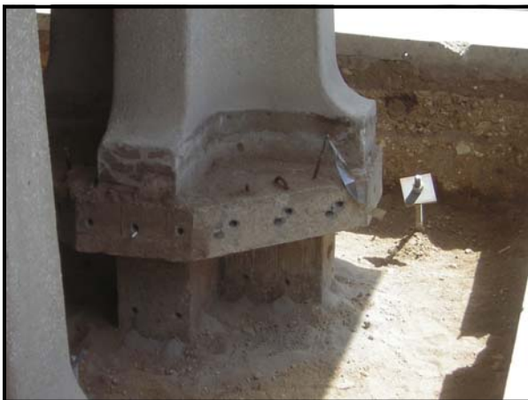
Figure 2. Construction process used for installation of helical soil anchors (A) surrounding soil excavated around the column (B) helical soil anchor installation (C) proof testing helical soil anchor (D) compaction of soil surrounding the column (E) drilled holes for installation of epoxy coated anchors, and (F) rebar reinforcement before concrete is poured.
