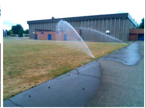
NW Elevation View locker room on bldg C same type as bldg A
