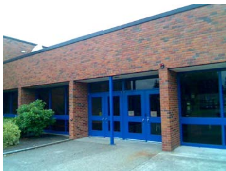
S Falling Hazard
