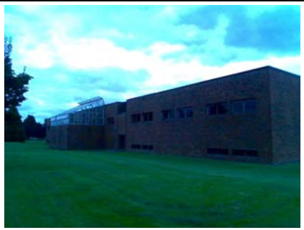
SW Elevation View
