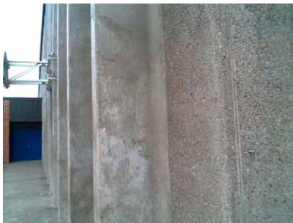
NW Primary Structural Type Caulked edge.
