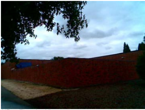
NE Elevation View Wall around mech/loading dock area.
