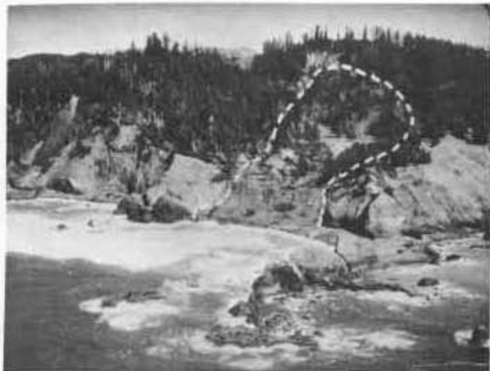
Figure 1. Aerial view of Ecola Park showing 1961 landslide (outlined in white). Ecola Point and Sea Lion rock in right foreground.
