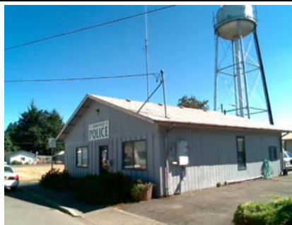
SW General Site
