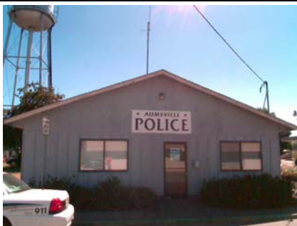
W Building Name
