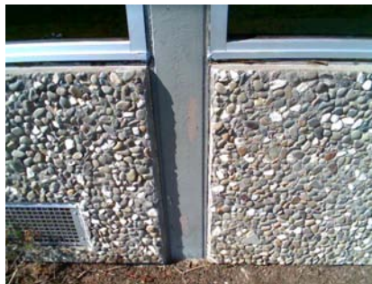
N Primary Structural Type Steel columns with some concrete at base wood roof beam at the top of the steel.
