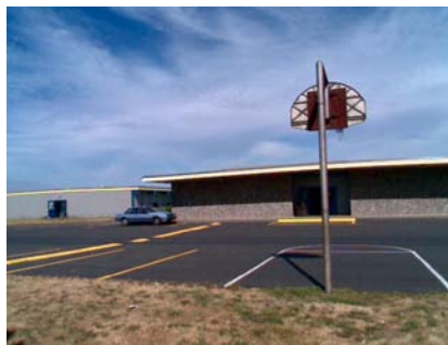
NE Elevation View
