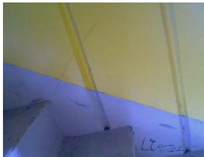
NE Primary Structural Type Solid Concrete seams no caulk
